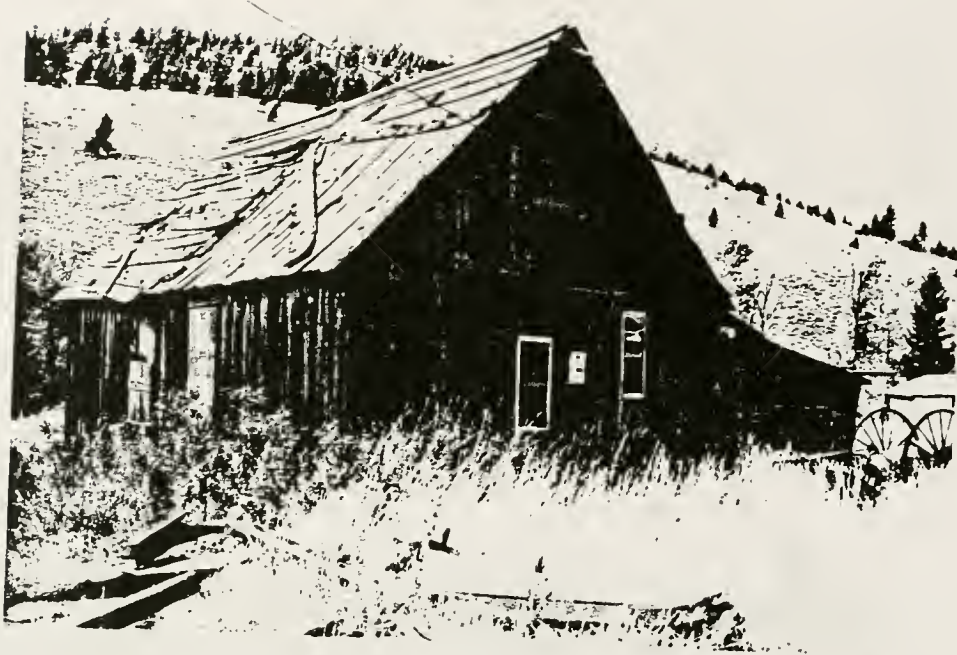
Figure 209. Structure #90, northwest view.
